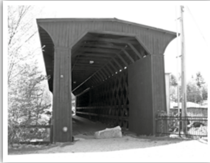
The Contoocook Railroad Bridge
